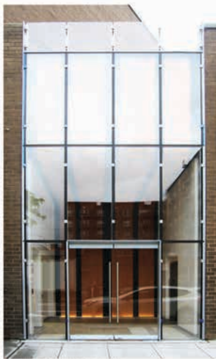
FLUSHING PLAZA/ MUSS DEVELOPMENT
